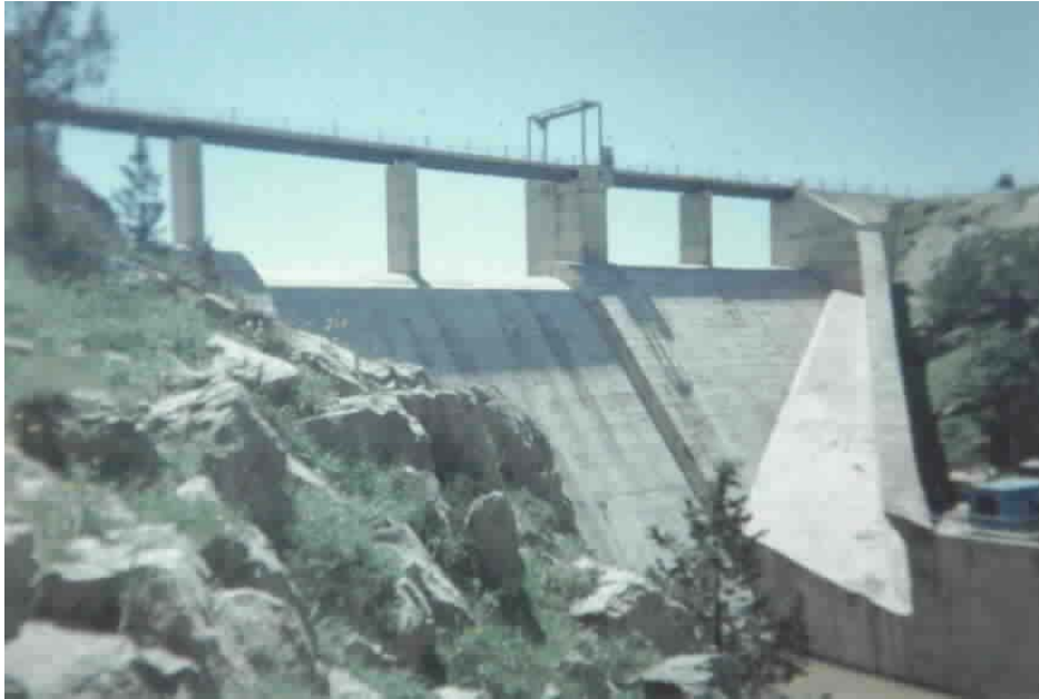
Photograph 1: General sight of the dam of the Hammam-Grouz
